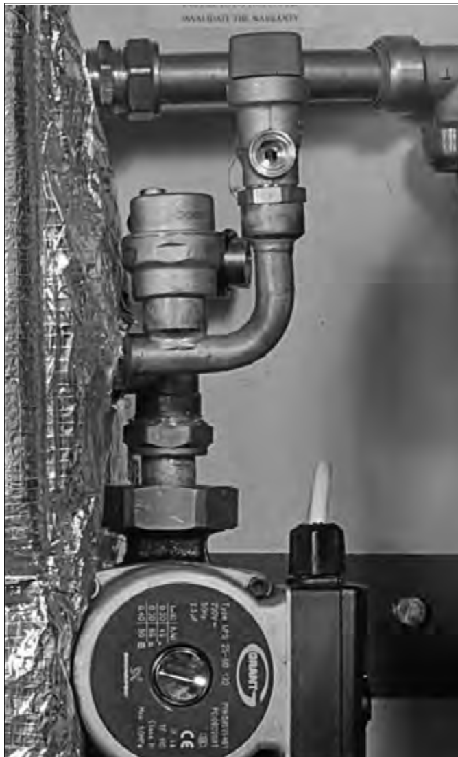
Figure 4-3: Removing flow and return pipe
