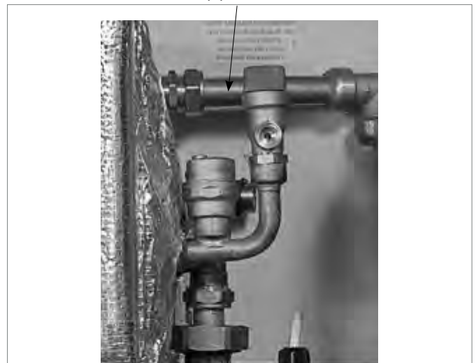
Figure 4-8: Re-fitting flow and return pipe
