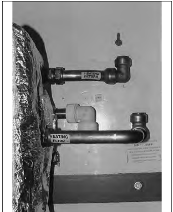
Figure 5-1: Non system boiler flow and return connections
