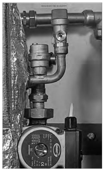
Figure 4-2: Removing flow and return pipe
