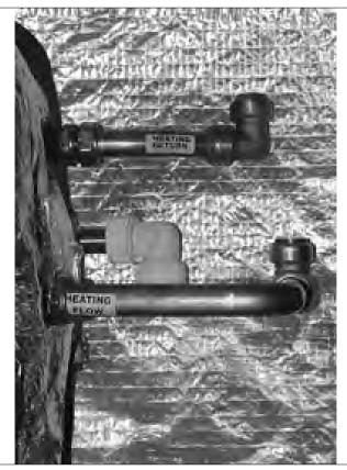
Figure 5-1: Non system boiler flow and return connections
