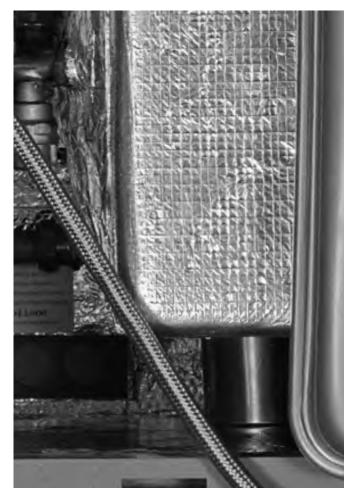
Figure 10-1: Boiler with front panel removed
