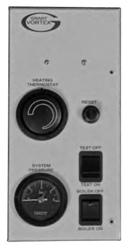
Figure 10-2: Boiler controls
