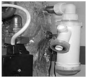
Figure 6-2: Condensate trap
