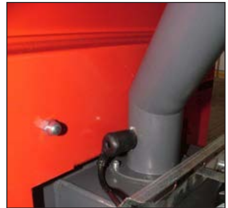
Figure 6-1: Location of pellet feed tube thermostat
