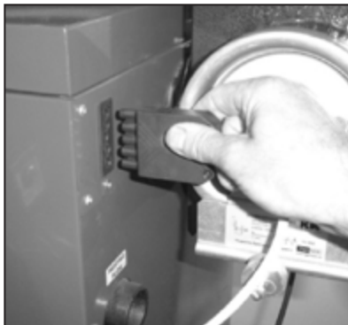
Figure 11-2: Disconnecting fan/solenoid 5-way plug
