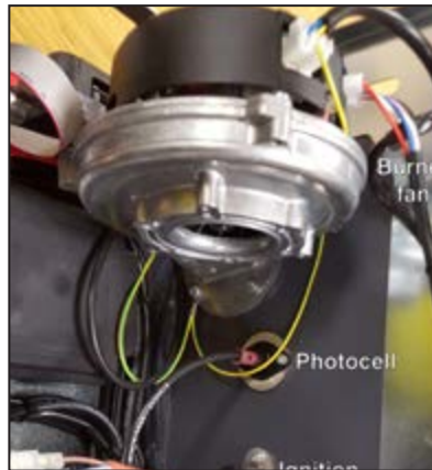
Figure 11-15: Burner fan, photocell and ignition element (6-26 and 9-36kW models)
