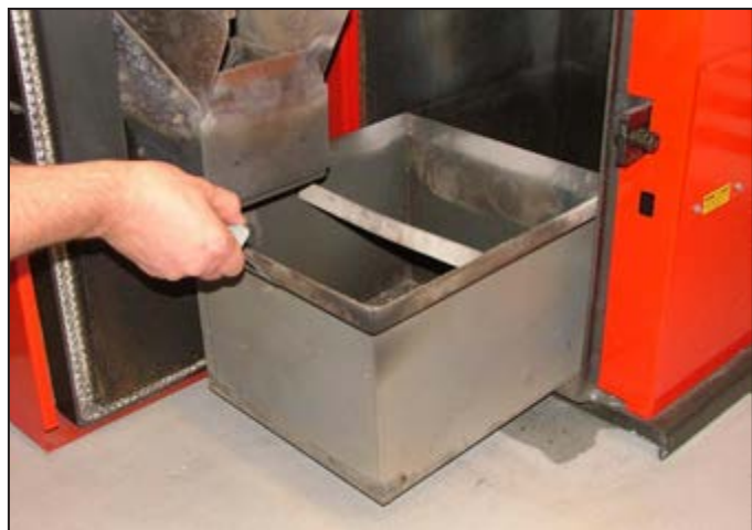
Figure 10-6: Removal of ash pan from boiler
