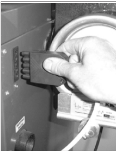
Figure 4-4: Flue fan/solenoid valve plug connection
