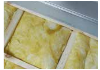
Heat emitter plates on cross battens
