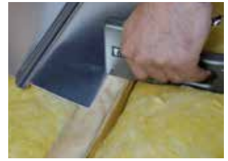
Fix plates to joist using staples
