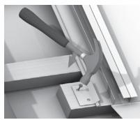
Figure 63: Securing Side Gutter Clips
