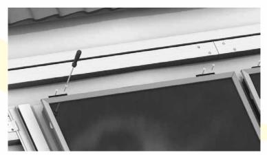
Figure 71: Fixing of the Top Brackets
