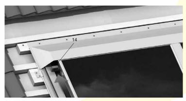
Figure 74: Fitting Foam Block (14)
