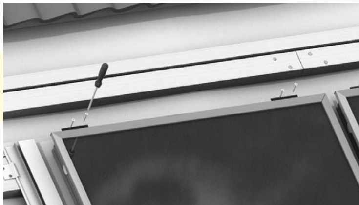
Figure 71: Fixing of the Top Brackets
